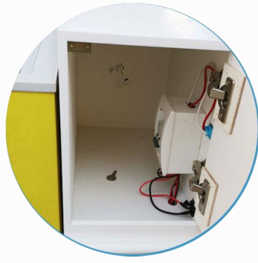
Side cabinet on part storage switch
